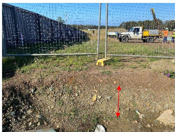
Looking east at excavated profile on boundary of Lot 208 and 400 exposing topsoil overlaying site won gravel fill to 0.7m.
