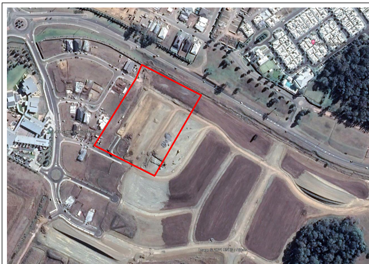
Plate 1: Satellite image dated July 2021 obtained from Google Earth that illustrates the site location and setting. The approximate site boundaries are outlined in red. Stage 1 was modified by site regrading earthworks including cut of up to 5m and fill of up to 1m.
