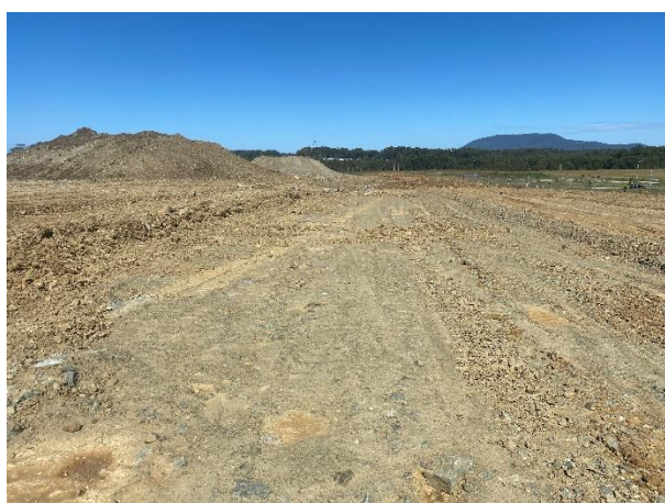
Replaced crushed rock fill in over-excavation area in Lot No's 231 to 237.
