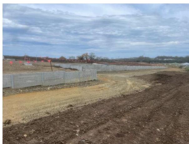
Looking east towards the continuous retaining wall across Lot No's 216 to 223.
