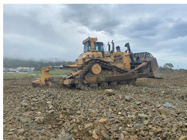
D11 bulldozer ripping weathered rock in over-excavation area.
